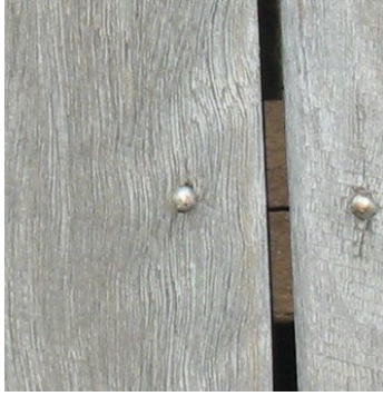
Split joist from stainless steel gun-nails driven in line
