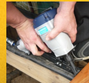
Position Gun Into Grooved Decking & Shoot!
