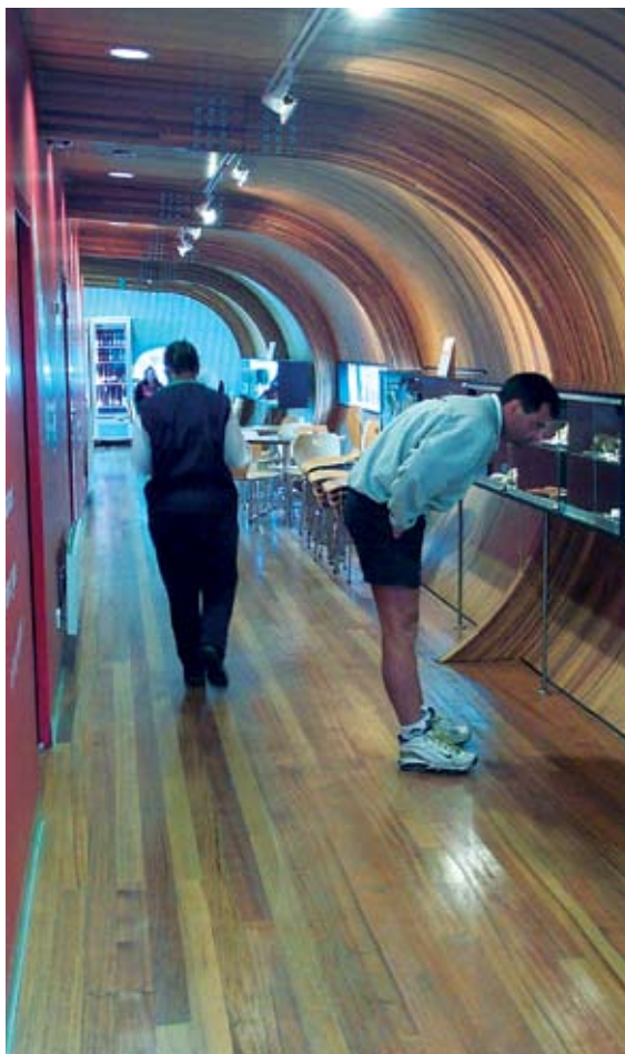
Beauty in carbon storage - curved beam and lining in the corridor of Dismal Swamp Visitors' Centre owned by Forestry Tasmania in Smithton, Tasmania
